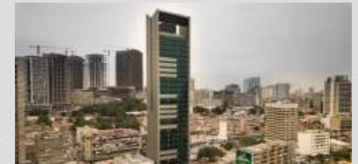
Residential and Office Tower, IMOB Luanda – SAVE 4M€ (7400 ton. CO2)
